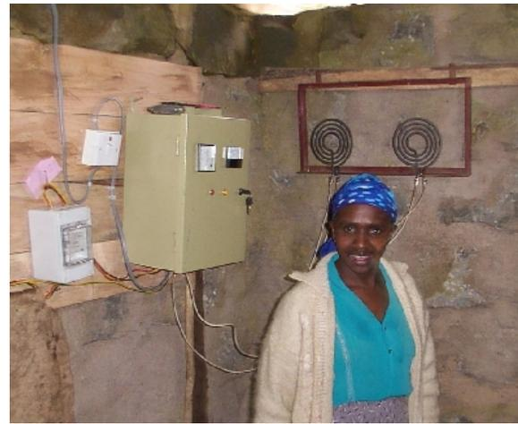
**Two 1.8kW cooking rings have been used as a ballast load. An RCD (left) improves consumer safety by minimising the risk of dangerous electric shocks.**
